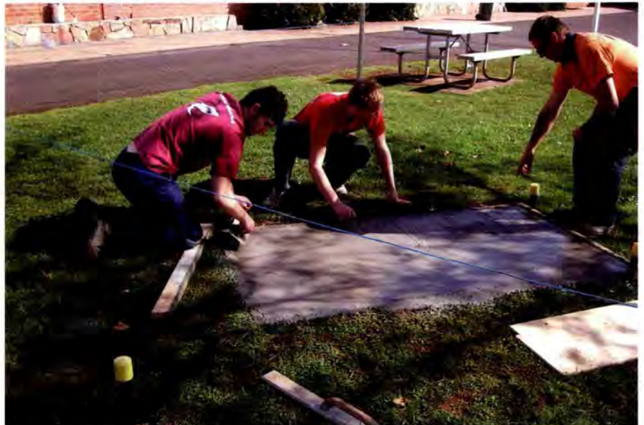
Above: Under the supervision of groundsman John Clousen, VET Construction students Zac Hislop and Jeremy Turner lay the concrete footings for some much appreciated outdoor seating on the bank near the Harcombe Centre.
